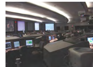
2 Operational Control Centers
