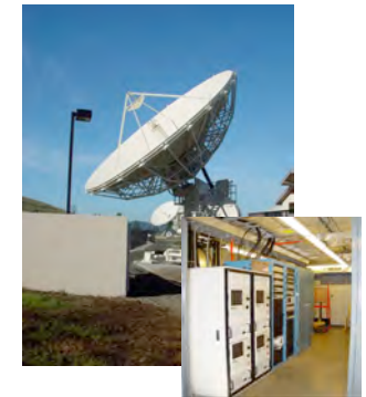
4 Ground Earth Stations
